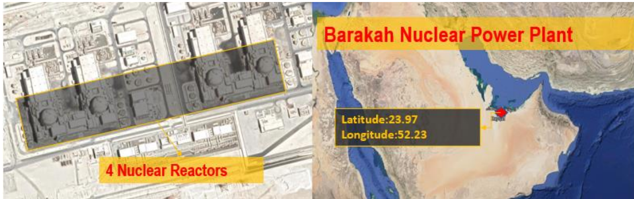
Figure1. Satellite map of Barakah nuclear power plant in the United Arab Emirates
