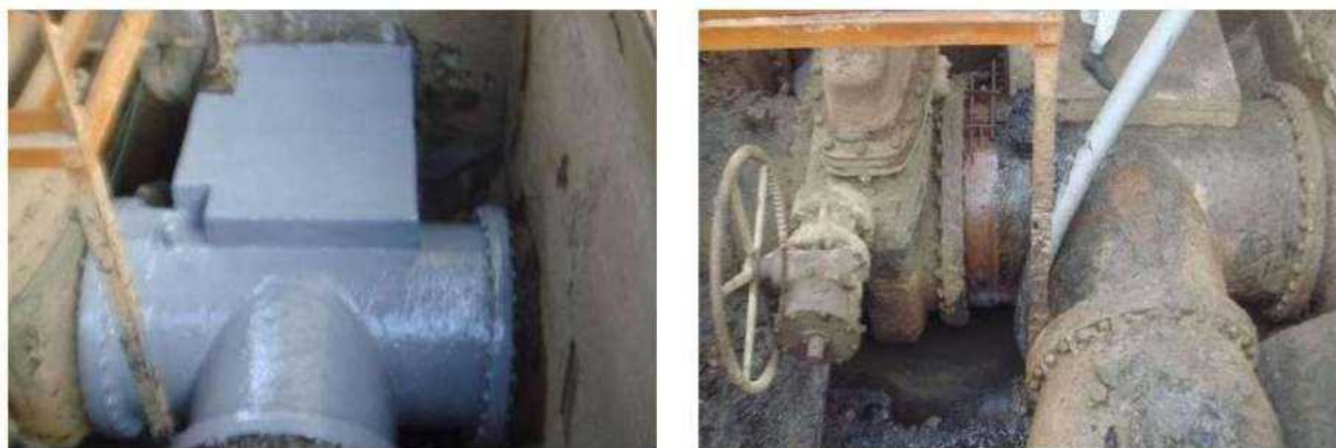
Fig 5. Using of nickel nano-composite coating in water supply system in PWL system
