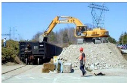
Fig. 3. The strategy: deferred dismantling, also called secure enclosure
